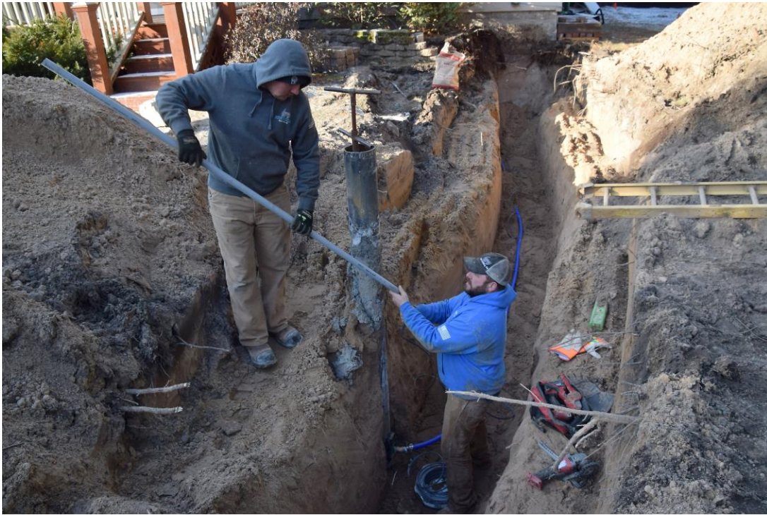
Digging trench and installing pipe to connect well to house
